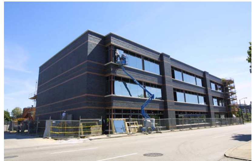
Business incubator under construction
