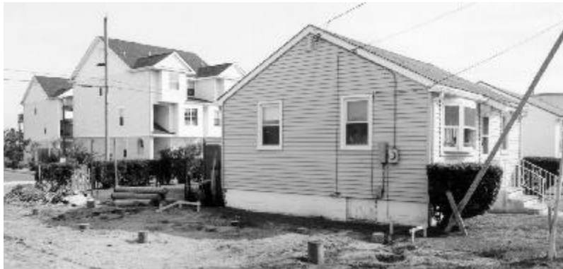
NEW STRUCTURES BUILT BEHIND SMALLER VERNACULAR HOMES IN CAPE MAY, N.J.
